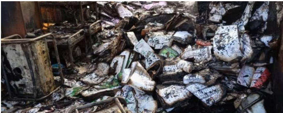
INEC facility after attack
